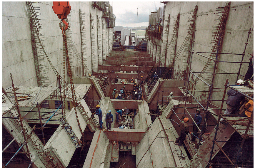
A coal bunker under construction at the Sasol 2 complex at Secunda.
